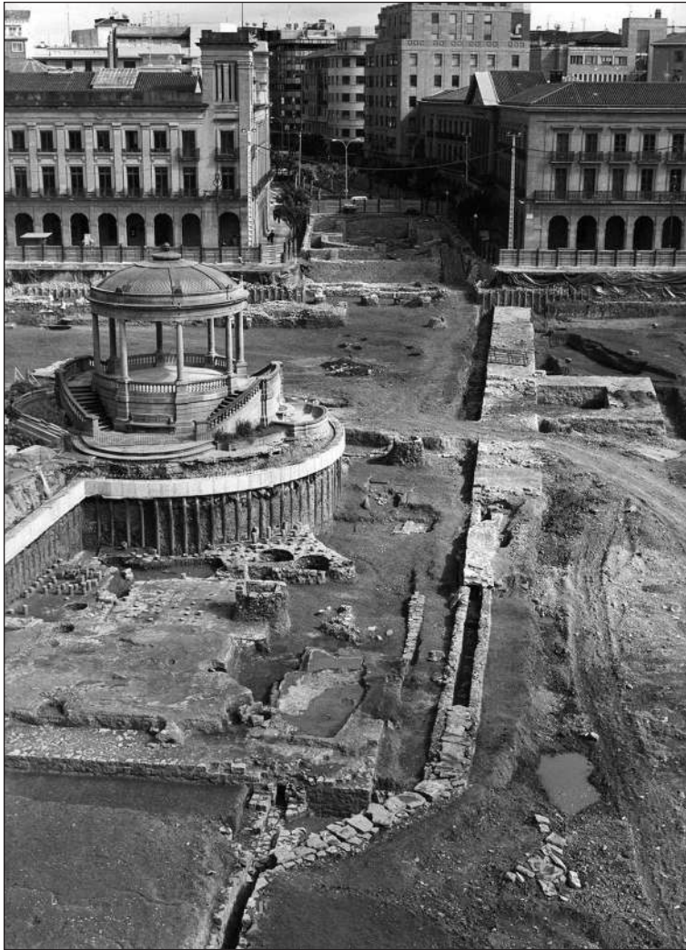
■ Figure 5. General view of the water draining system from the north.
